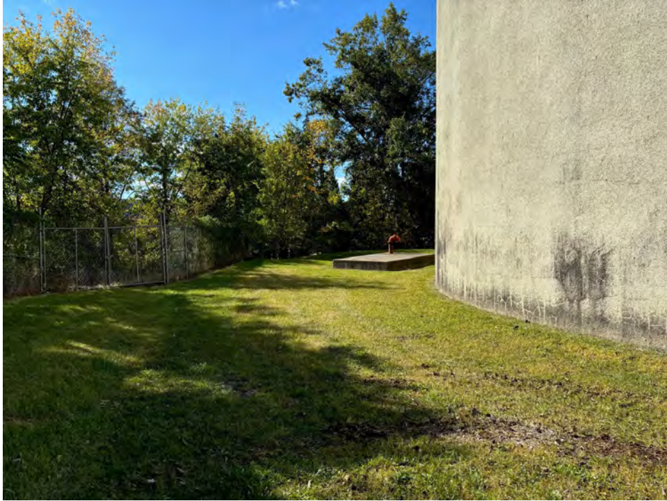
Photo 7. View from north of the project area facing southwest
