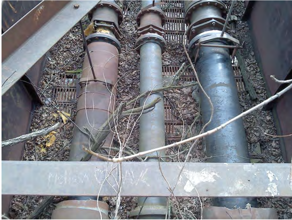
View looking at piping on pipe bridge from west side
