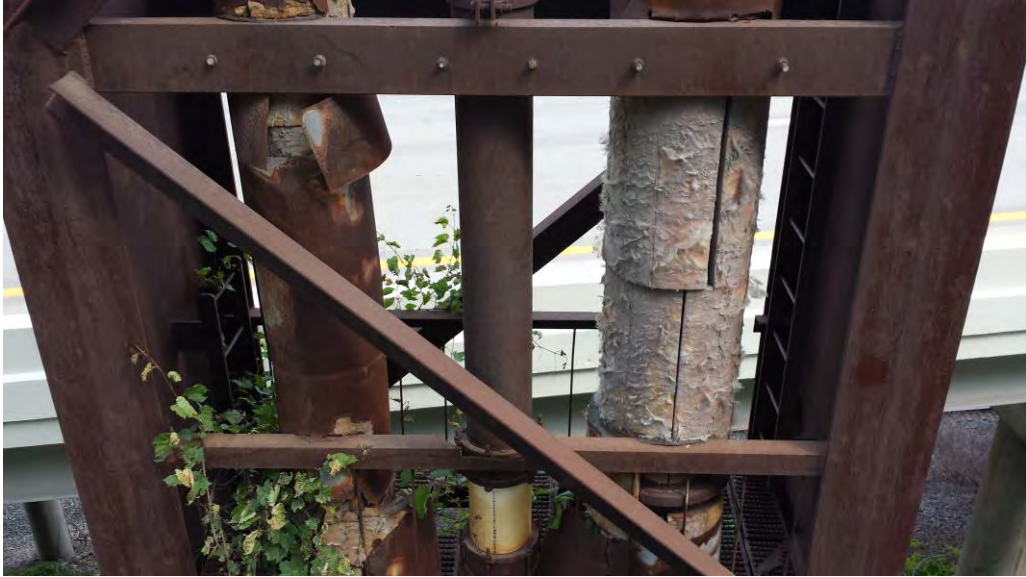
View looking at east side/bottom of pipe bridge & piping
