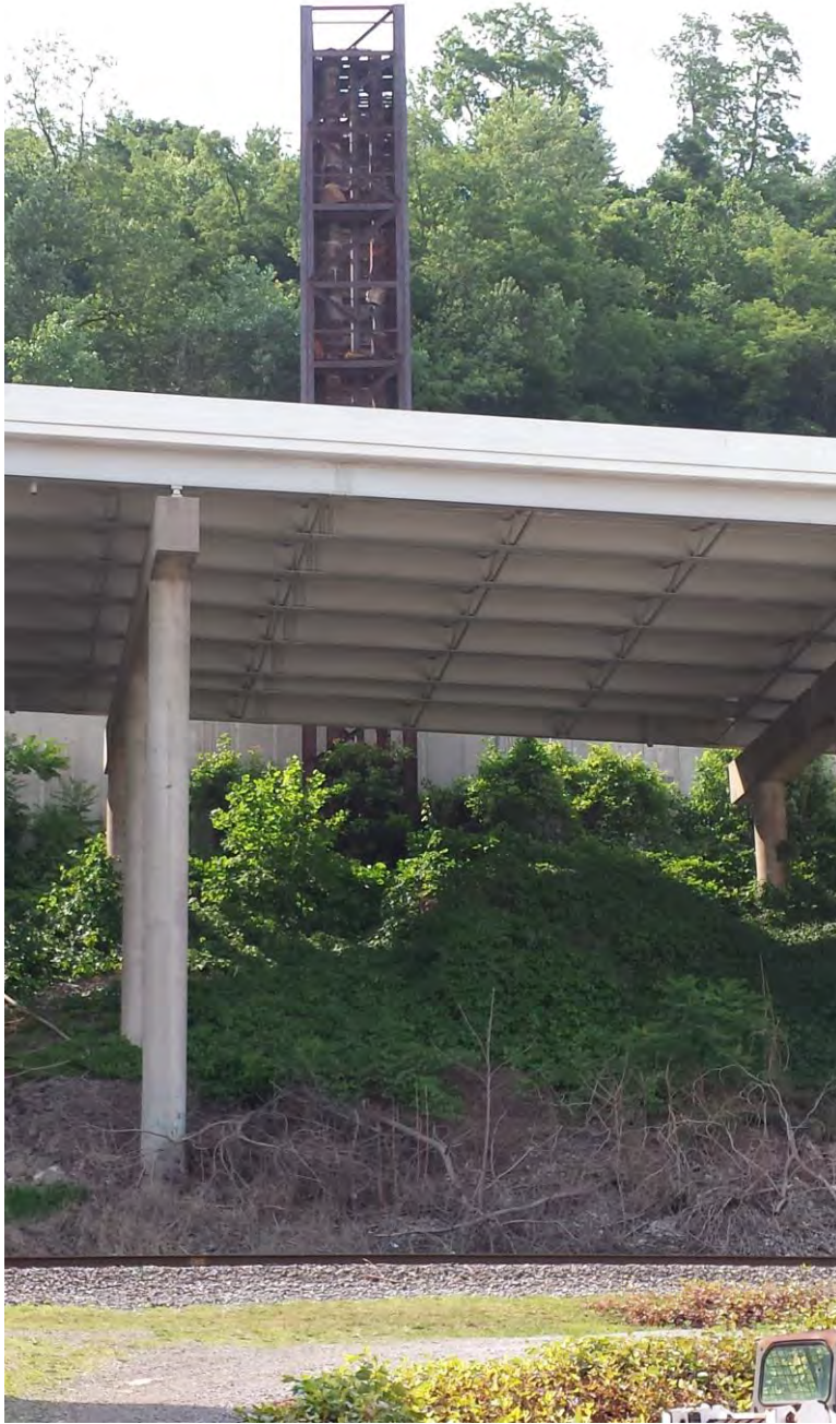
View looking at east side of pipe bridge from River Road
