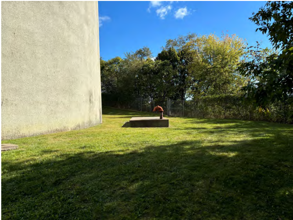
Photo 6. View from south of the water tower facing northeast
