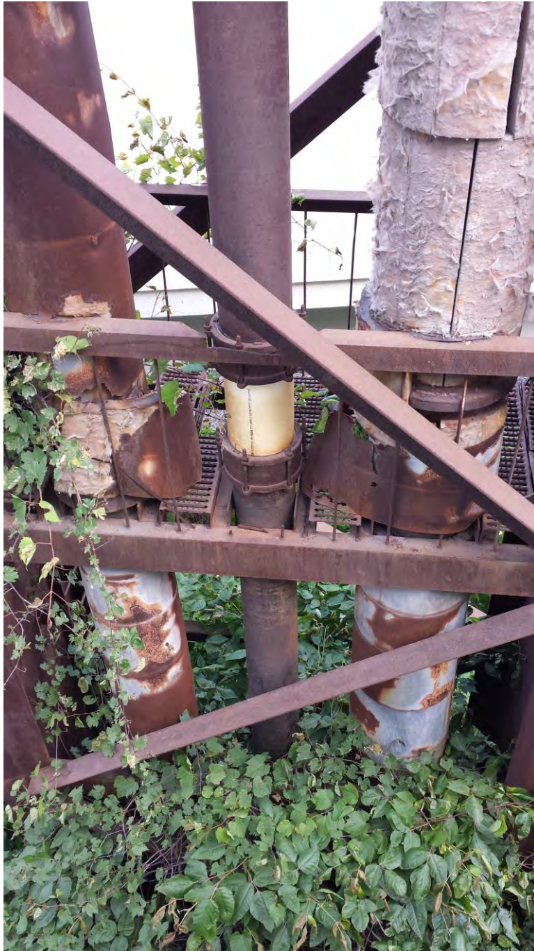
View looking at east side/bottom of pipe bridge & piping
